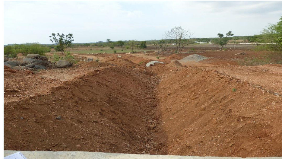
WORK UNDERWAY FOR CANAL IRRIGATION
